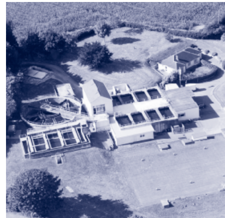
Augrès Water Treatment Works
