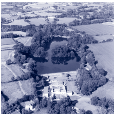
Handois Water Treatment Works
