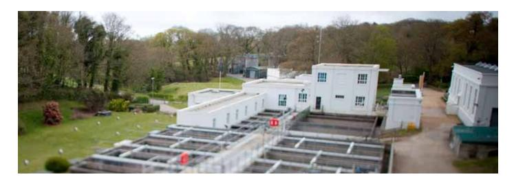
All of the water supplied by the company is treated at one of it's two water treatment works located at Handois and Augrès. Both sites are situated at approximately the same height above sea level so as to facilitate the movement of water into the distribution system.
