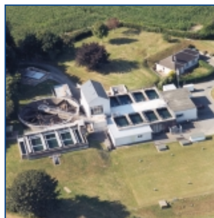
Augrés Treatment Works
