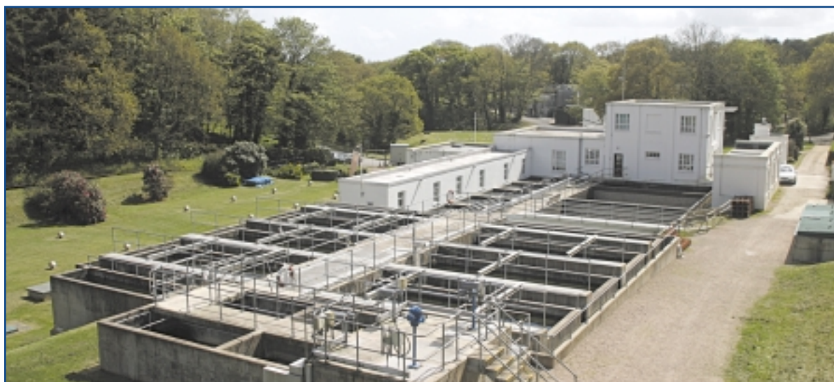
Handois Treatment Works
