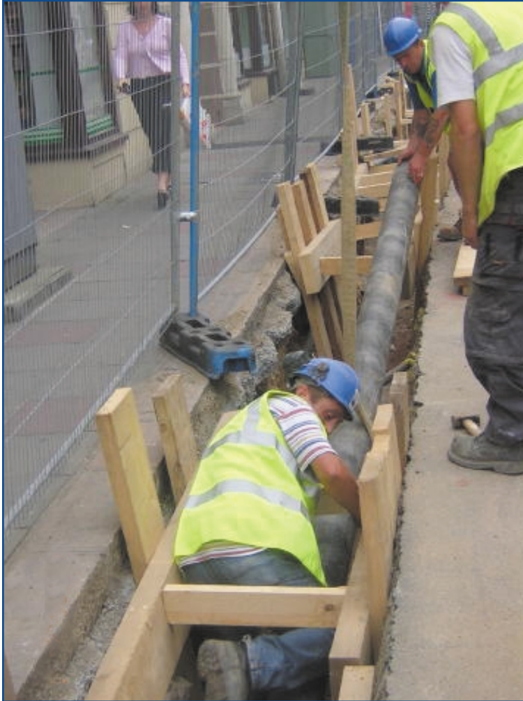
John Le Guilcher, Foreman Mainlayer (in the foreground) and his team laying a replacement 150mm diameter water main in Union Street, St Helier
