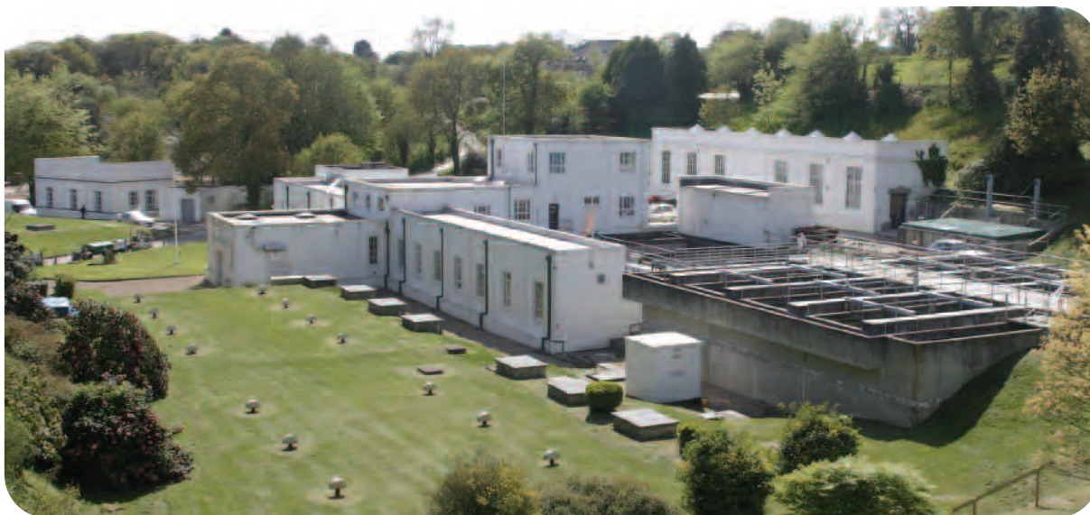
Handois Water Treatment Works
