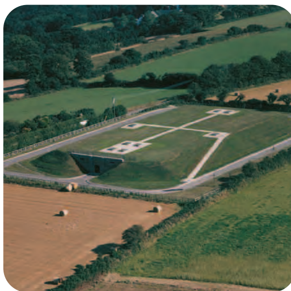
Les Platons treated water service reservoir
