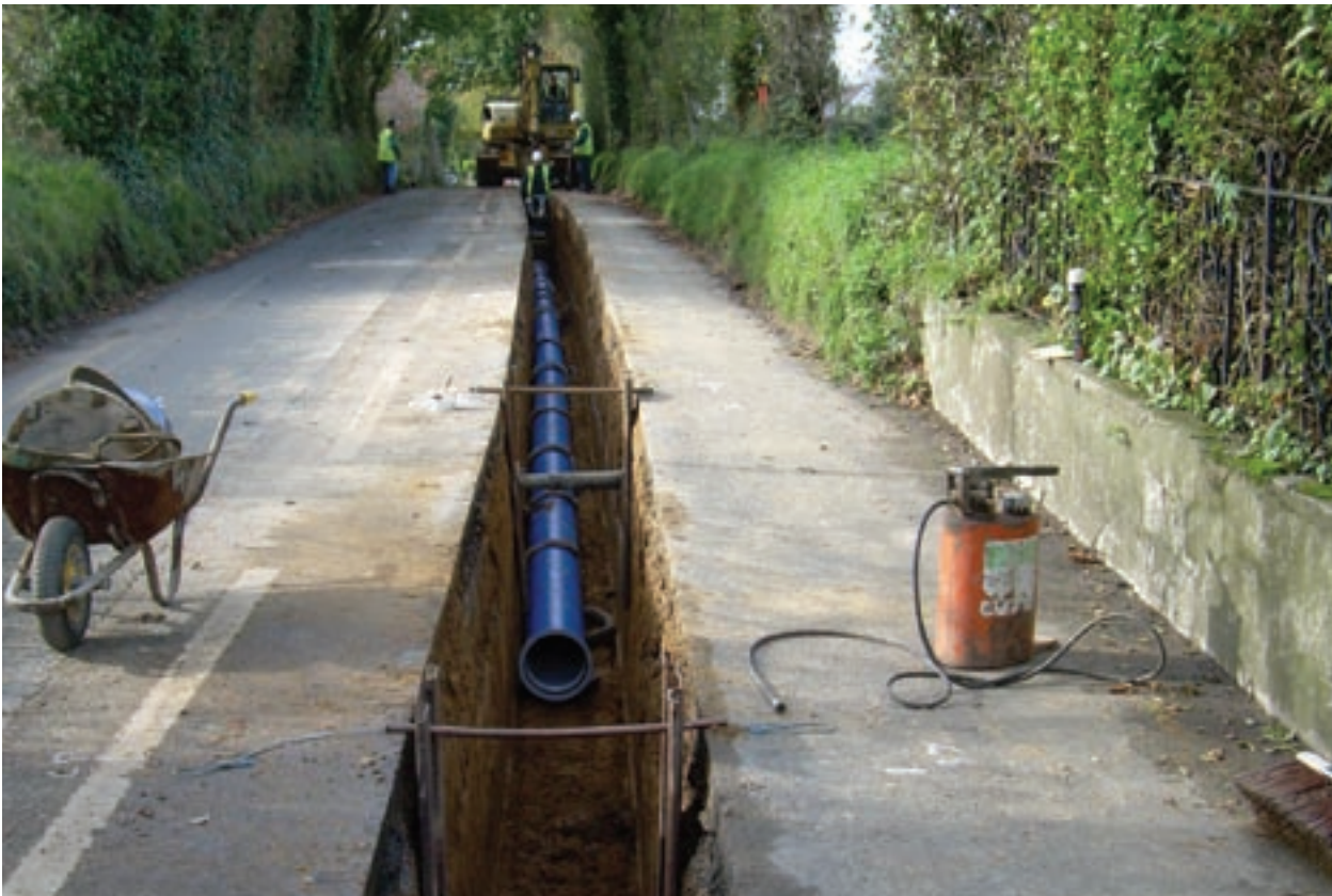
Laying the 300mm trunk main in Trinity.
